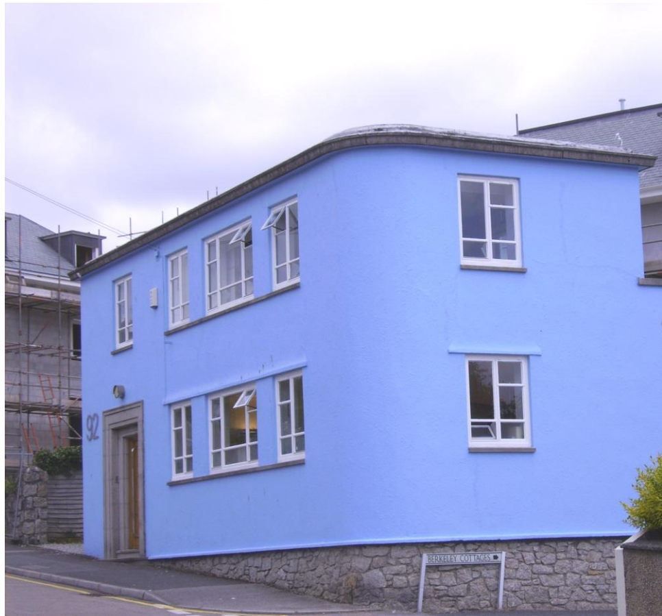
Figure 3: Until recently, occupied by a graphic design firm, this was the western headquarters of NDLS in Cornwall at Kimberley Park end of Trevethen Road, Falmouth.
