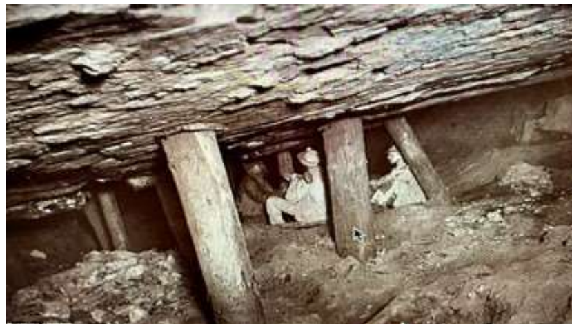
Figure 15: Pit Props in a nineteenth Century Cornish mine Source: J.C. Burrows c. 1890
